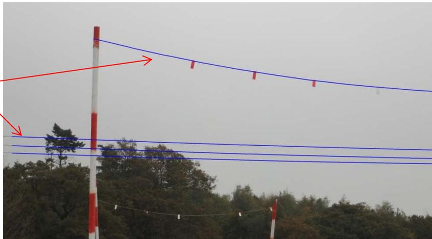
The guys were carrying out an excavation between a set of goal post markers that identified the position of the overhead cable, but thought that they would not hit it despite the cable being below the level of the goal posts. Clearly this proved not to be the case and when Paul hit the cable with the excavator both Andy and Clint were extremely lucky not to be killed.
